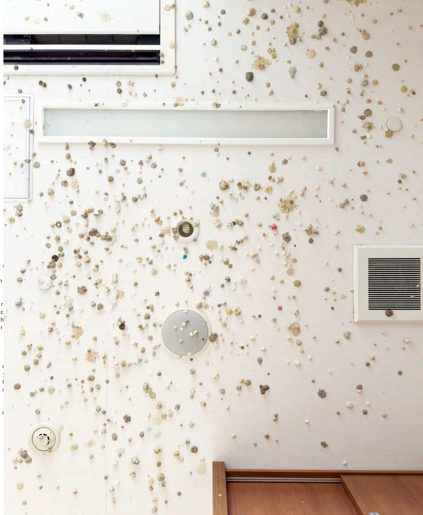
W Ĩ Ł U Ś I U R X Ů Documentation photo of the ceiling at Kumi Gakuen Taken on November 10 , 2025
